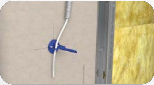
1. Adhere the Adhesive disc to the Cable holder and peel of the protective film. Fasten the Cable holder to the dry wall and feed cables or conduits through the brackets.
