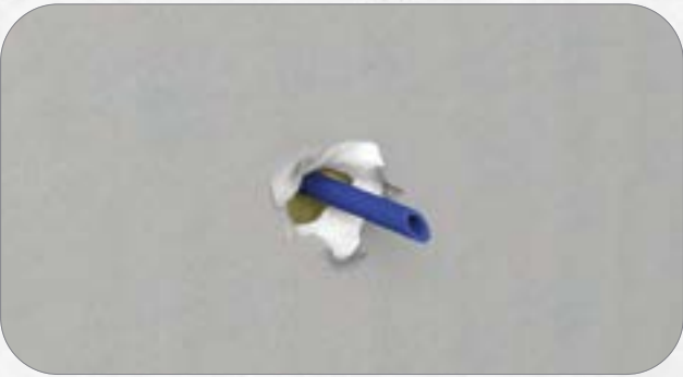
2. Push an angled mandrel through the second plasterboard or tap in a hole with a hammer beforehand.
