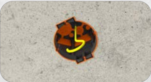
6. Ceiling installation: Ceiling hook holder according to EN 60670.
