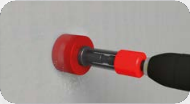
4. Place the box mill in the centring hole and mill out the hole.
