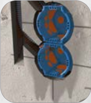
3. With a plastered wall, simply break off the plaster stop and insert the box fully.
