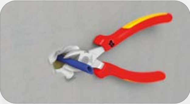
3. Pinch off the Cable holder flush with the wall.
