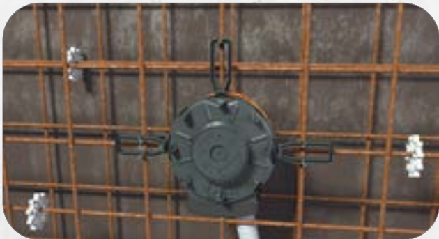
3. A third wing can be mounted for additional hold.
