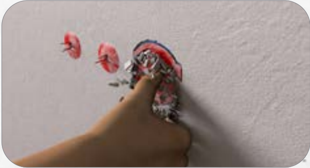
6. Signal pins ensure quick location. Push the cover in with your finger or screwdriver. When it pops outwards, a clean contour is created without offsets in the plaster. Then remove the cover.
