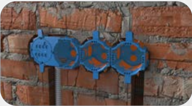
2. Insert the boxes up to the plaster stop. A standard-compliant and flush-mounted installation is thus ensured.
