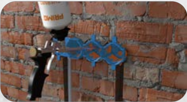
4. Use the Foam pistol to break out the predetermined breaking point in the rear of the box and inject the foam until the box is completely enclosed. After 30 minutes, the foam is cut-resistant.
