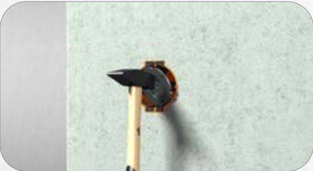
1. After concreting, the cover can be opened with a hammer blow.
