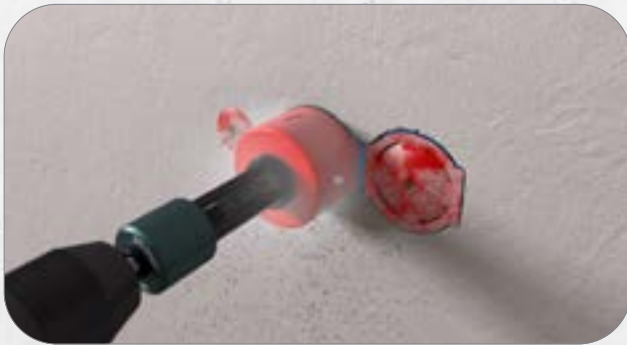
7. Alternatively, expose the plaster cover with a 68 mm holesaw and remove it.
