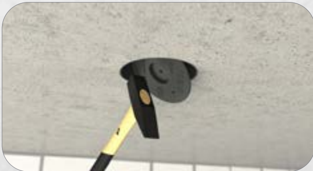
5. Open the Front part with a hammer blow after demoulding.
