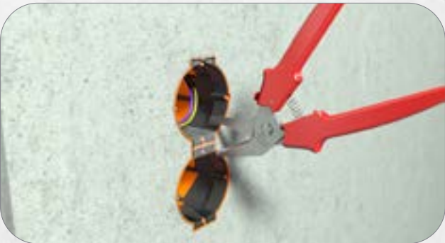
4. If necessary, remove the SCS connecting web effortlessly with the Primo Box cutter.
