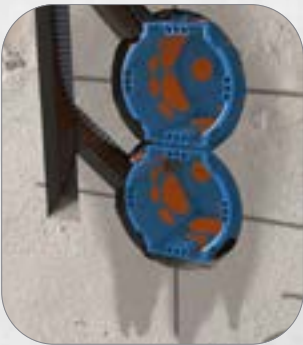
3. With a plastered wall, simply break off the plaster stop and insert the box fully.
