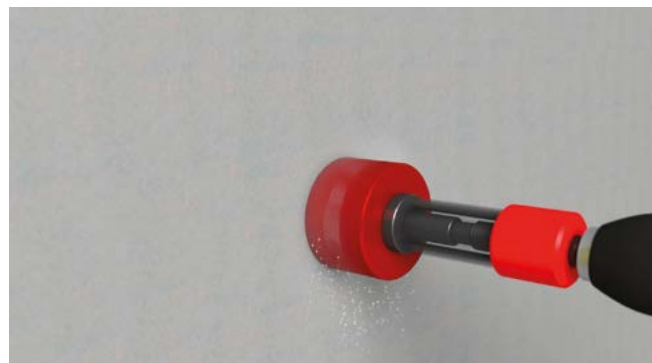
Mill out the hole with the holesaw.
