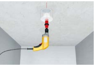
The individual opening is drilled out with a holesaw ...
