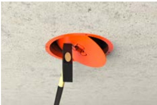
Knock in the Ventilation sleeve from below with the hammer.
