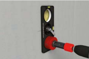
Then saw through the existing hole inserts.
