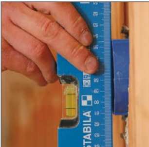
... so that it protrudes about 1 cm from the brickwork.
