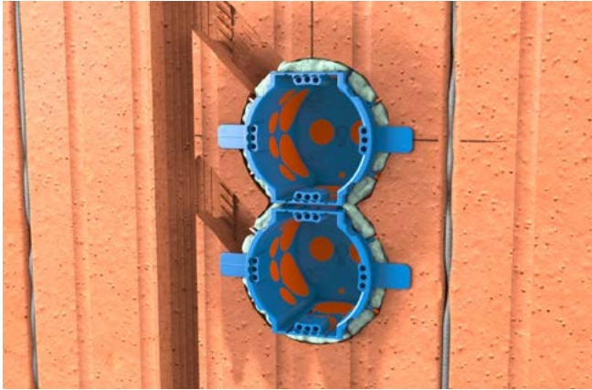
Break out the remaining web when the foam has hardened.
