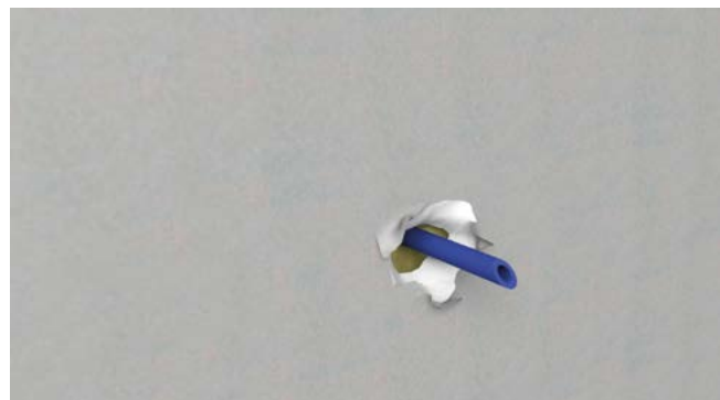
... make a hole with the hammer. Push the mandrel through – it serves as a centring aid.
