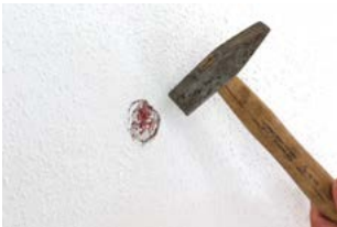
Tap lightly on the plaster cover with the hammer.
