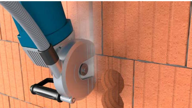
Mill a slot with the brickwork groove milling machine along the drill holes.
