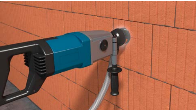
Mark the first box and drill with 82 mm holesaw.
