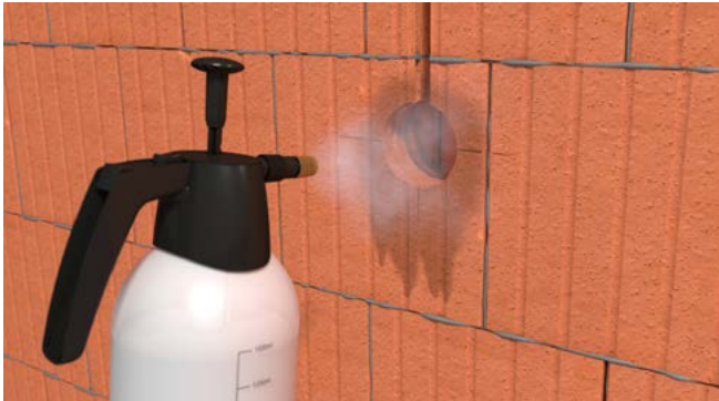
Moisten the hole so that the foam swells better.
