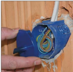
Push the Drill cover on.
