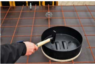
Nail to the formwork in case of cast-in-place concrete, or glue to the
