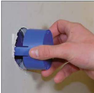
Push the upper part of the box on and push in until flush
