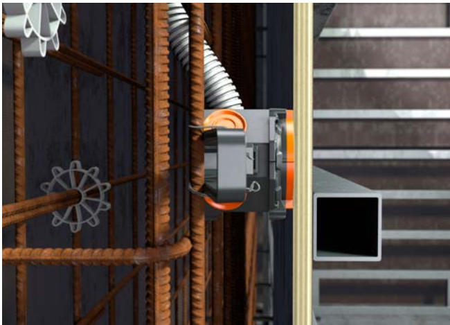
Flexible Wings adapt themselves to the respective concrete cover. Concrete covers of 20 – 40 mm or 40 – 60 mm. Concreting can take place after placement of the opposing formwork.
