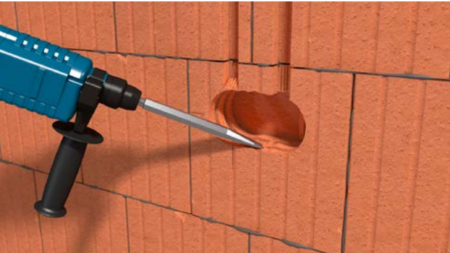
Chisel out protruding corners.
