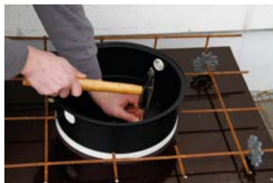
Nail to the formwork in case of cast-in-place concrete, or glue to the formwork table in the precast plant.
