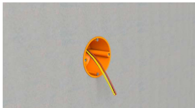
Mount the Cavity wall box and install the built-in device/socket.
