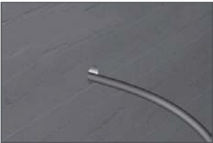
Drill 35 mm hole with a slight downwardly/outward inclination; pre-wet the drill hole and insert the cable/pipe.
