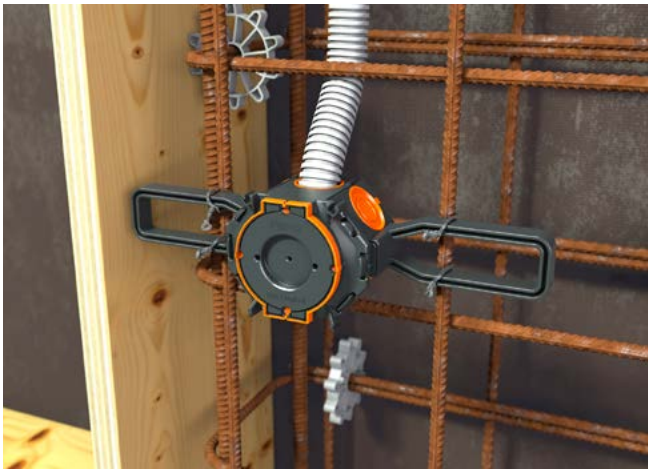
Fasten the wing to the steel reinforcement with wire.
