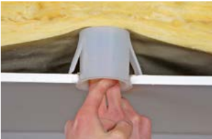
Push the Protective cap into the drill hole.
