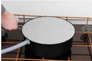
Insert conduits/cables and fasten the stable sheet metal plate with the cable tie.
