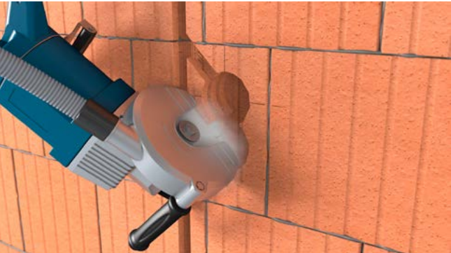
Variant 2: Mill the slot into the box hole.
