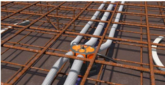
Lay the second steel reinforcement.
