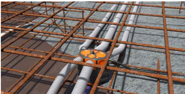
The Membrane box can be cast in concrete.
