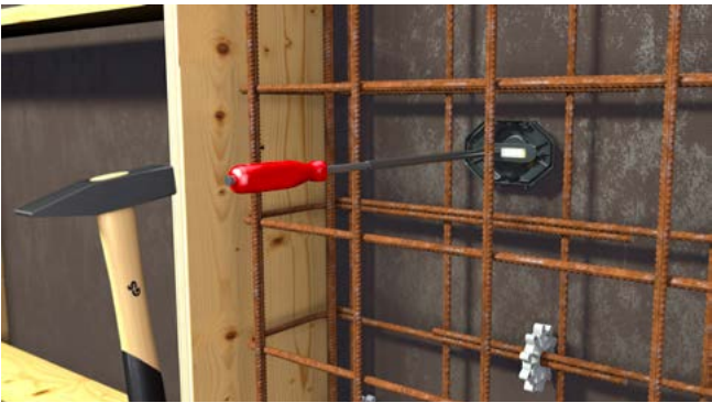
Align with the help of the integrated spirit level and nail on.
