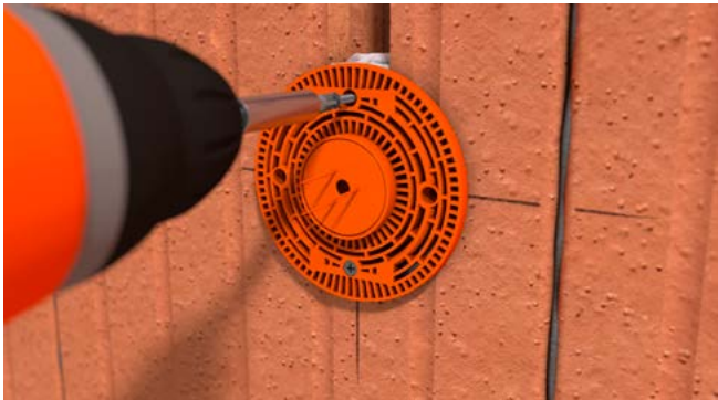
Push on the Equipment carrier and fasten it with 2 screws.
