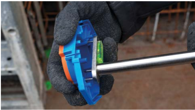
Pick up the cover with 60 mm holding pins.
