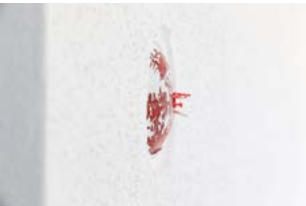
After plastering, the plaster cover stands proud.
