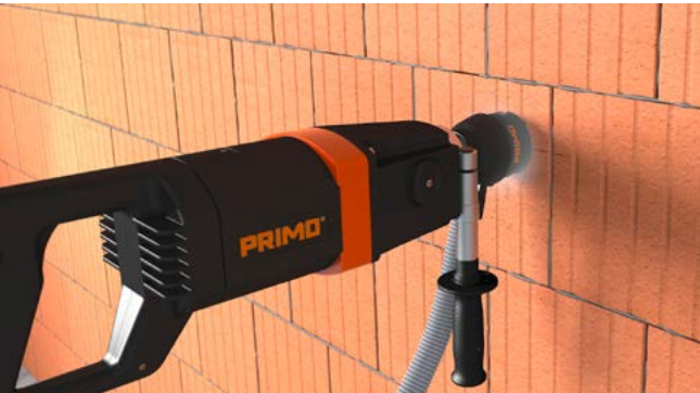
Mark the first box and drill with Ø 82 mm High-speed drill.
