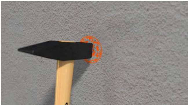
Carefully tap in the cover with Signal pins using a hammer.
