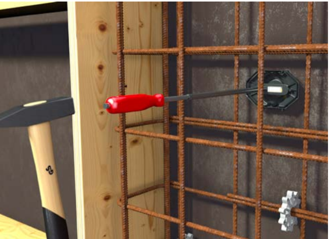
If the second reinforcement has already been attached, the cover can be positioned and nailed on using the nailer (P752).
