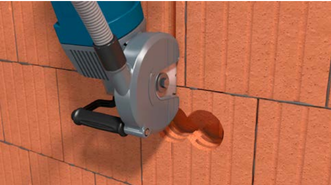
Variant 1: Mill a slot up to just before the box hole.
