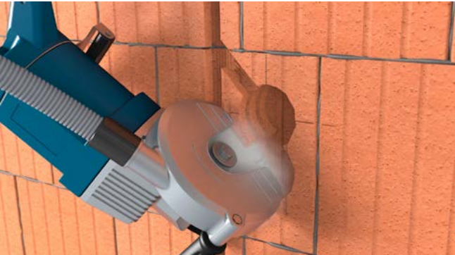
Mill the slot into the box hole.
