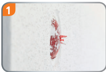
After plastering, the plaster cover protrudes.
